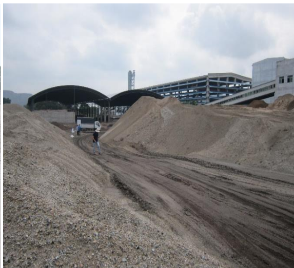
Figure 2. The dumping site of An Khanh TPP.
